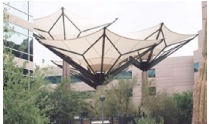
Upside down umbrellas that shade an employee plaza and collect rainwater for the plaza's landscaping. Source: Forgotten Rain L.L.C.
